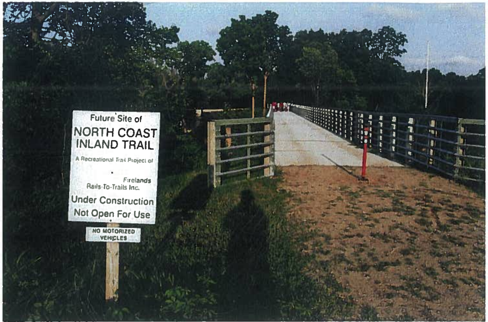
ABOVE: The new Rails to Trails bridge over the Huron River between Monroeville and Norwalk parallels the Wheeling & Lake Erie bridge. JAMES SEMON
