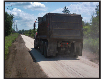
Joe Wilhelm and crew bring in truck loads of 9D crushed limestone for a smooth trail surface.
