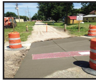
Spring posts are installed and smooth concrete aprons are poured at the roads.
