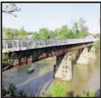
The Huron River Bridge is complete and will see through traffic soon!
